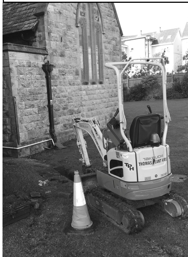
Work projects at St Paul's. ABOVE: the reflections in this puddle by the altar are pretty, but the water is bad news. A leak in the roof some thirty foot above will cost thousands to repair. BELOW: plant roots blocking the drains meant a complete rebuild of the system lasting two days and involving a completely new section of pipe.
